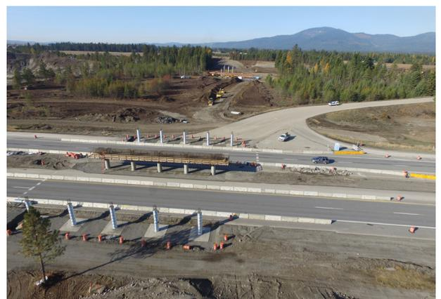
October 2019: Aerial view of US-95 and ID-53 intersection with new interchange foundation structure in place.
